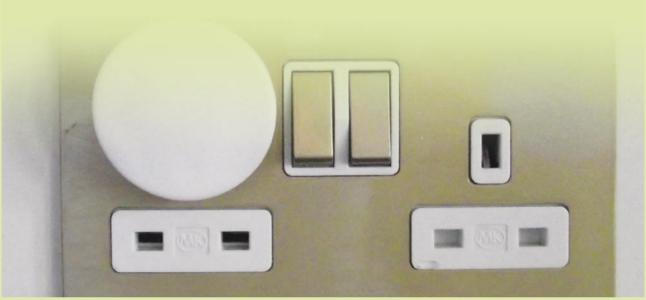
Figure 1 - Wrongly inserted socket protector.
