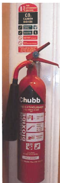
Figure 10 - A carbon dioxide fire extinguisher.
