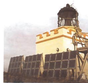
Figure 10 - Lighthouse on Brough of Birsay, Orkney Islands Solar panels useful even this far North!
