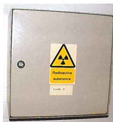
Figure 1 A radioactive source cabinet – stock should now be checked every month except in the summer holidays.
