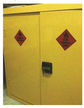
vi) Flammable cabinet. A fire resistant, lockable cupboard which for safety reasons should be located as far away from the entrance to the store as possible should also be provided. If the chemical store has the requisite 30 minutes fire resistance then there is no absolute need for a flammable cabinet though it might be advisable for some of the more highly flammable substances. (It is also possible that insurance companies might insist on it).
