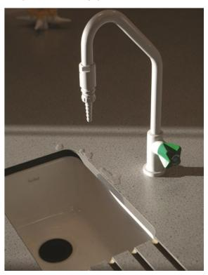
sink and the tap. A length of pipe attached to a tap means that it is possible for water in the sink or drain to flow backwards into the tap.
