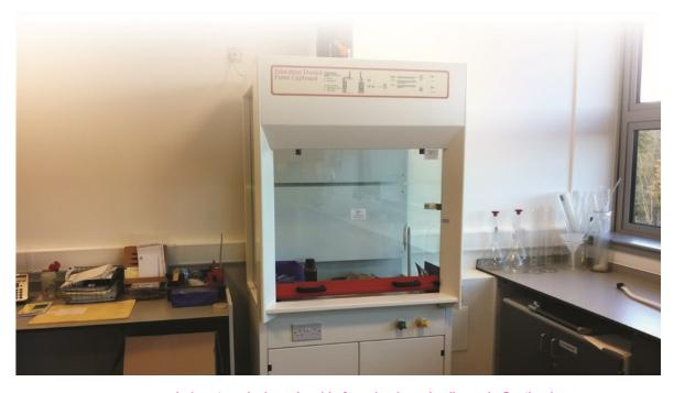
Fume cupboards should not be installed near doors or in the corners of rooms where air turbulence will affect their performance. Fume cupboards and room extractor fans should be on separate electrical circuits.
